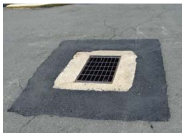
Catch Basin Top Repair
