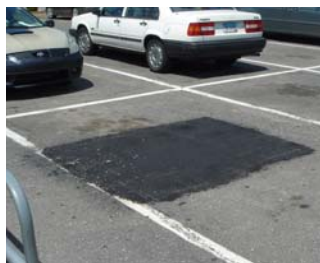
Pot Hole Repair
